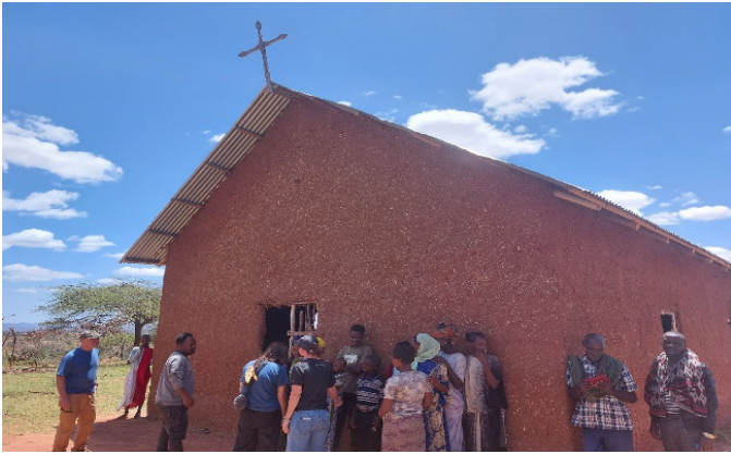
This church was recently constructed in a community where a drilled well was installed. The walls are a composite of chopped straw and mud, with green sticks as reinforcement around window and door openings.
