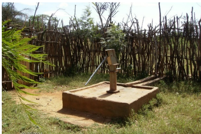
Typical wellhead and hand pump installation with barrier fence.
