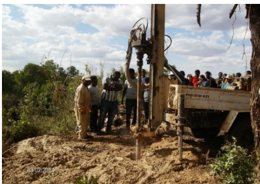
Well drilling is underway with a crew from LMI.
