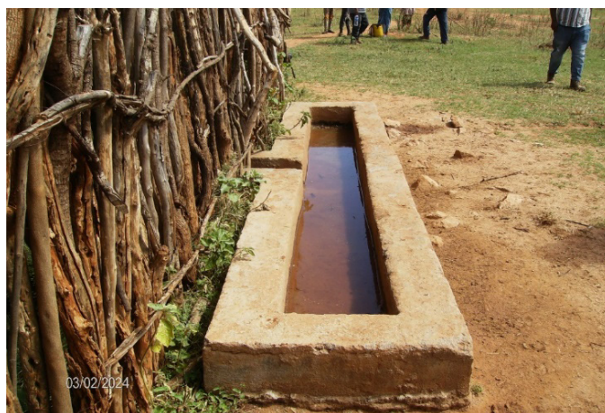
Overflow from the wellhead is contained and flows to a trough for livestock.
