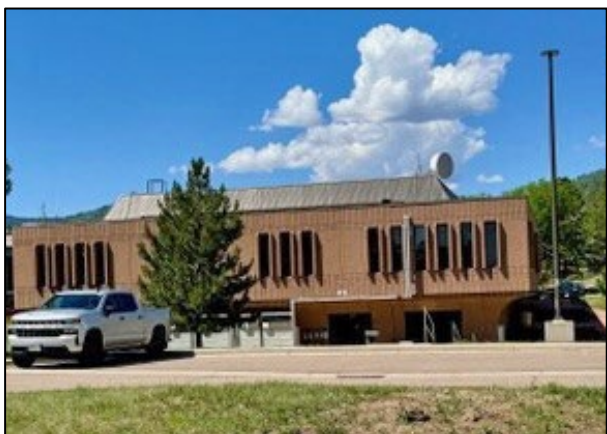
Operations Control Building
