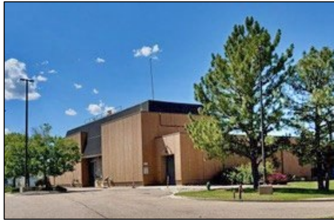
Chemical storage and feed building.
