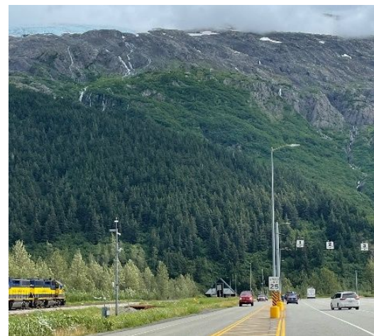
Train and cars at the tunnel access.
