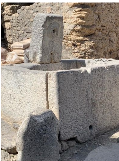
Typical street fountain in Pompeii showing spout stone, use wear, overflow, drain, and guard stone.
