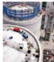
**Changi Water Reclamation Plant:** This 800-million-liter-per-day plant is currently in the final construction phase, having commissioned more than half the plant. CH2M HILL designed and is providing construction management and commissioning services for the plant.
