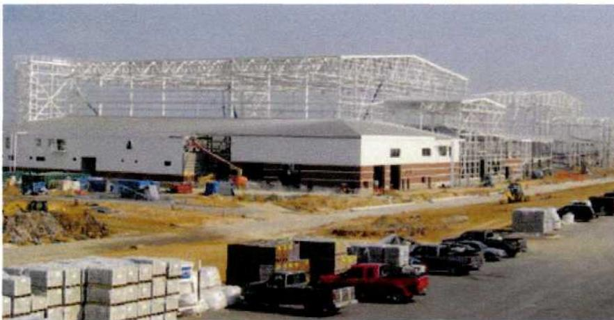
*This view shows recent hangar construction at Memphis International Airport, with the maintenance hangar in the foreground and the corrosion control hangar in the background.*
