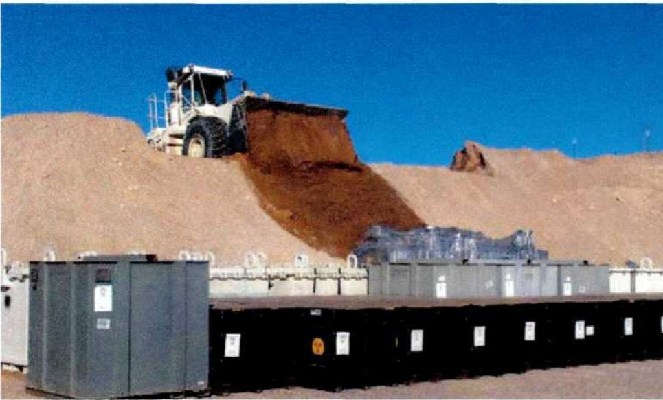
These containers hold the remnants of glove-boxes used in processing radioactive materials. Low-level and some mixed low-level waste is permanently disposed of onsite.
