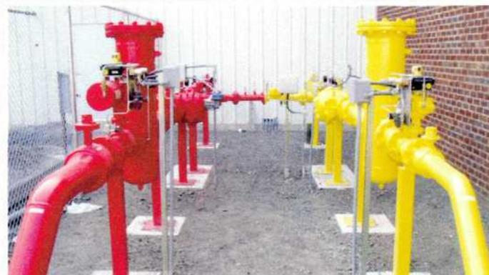
The blending station at the new plant blends natural gas as needed with landfill gas for use in the kilns.
