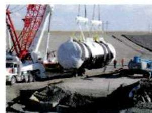
The four so called V-tanks were installed in the early 1950s as part of a system to collect and treat radioactive effluents from operations at Test Area North. U.S. DOE
