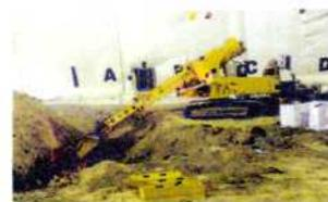
Since arriving in Idaho, CWI has exhumed nearly 1,900 cubic meters of waste. The waste contained high concentrations of volatile organic compounds and transuranic-contaminated materials.
