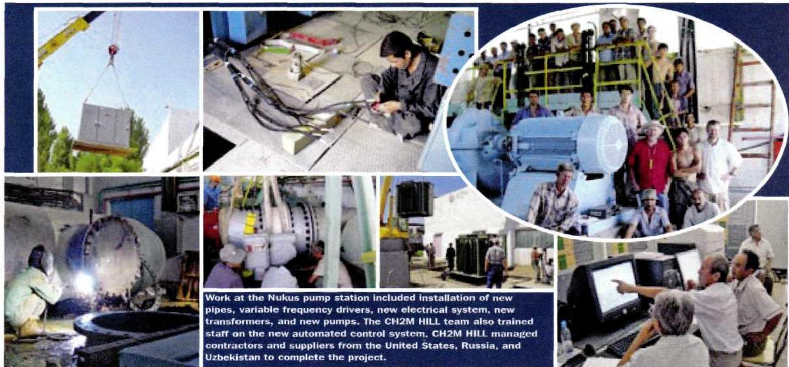
Work at the Nukus pump station included installation of new pipes, variable frequency drivers, new electrical system, new transformers, and new pumps. The CH2M HILL team also trained staff on the new automated control system. CH2M HILL managed contractors and suppliers from the United States, Russia, and Uzbekistan to complete the project.
