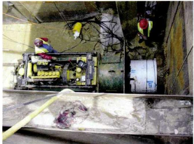
Construction workers install a pump and connecting pipeline leading from the Edwards Aquifer to the Carizzo Aquifer.
