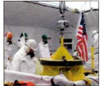
Crews pull the old pump from Tank AP-101, making room for a more powerful pump to feed waste to a treatment plant for glassification.
