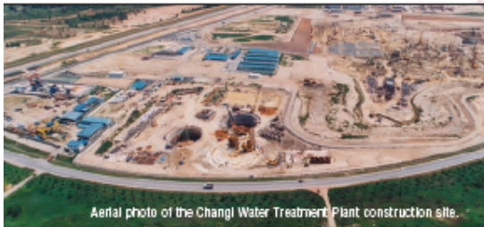
Aerial photo of the Changi Water Treatment Plant construction site.
