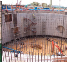
Pump station No.2 excavation and construction
