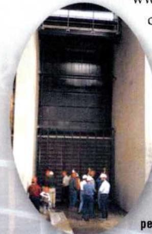
**Along the Sacramento River this 830 cubic-foot-per-second screen is 45 feet high and 250 feet long. CH2M HILL completed this project for Reclamation District 108.**
