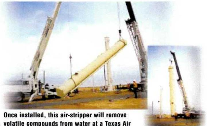
Once installed, this air-stripper will remove volatile compounds from water at a Texas Air Force base landfill. Remediation activities are among the many services CH2M HILL provides to the U.S. Air Force Center for Environmental Excellence program.
