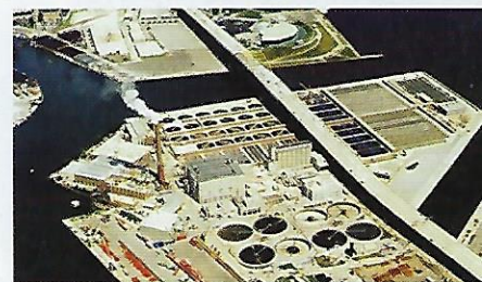
The Jones Island Wastewater Treatment Plant was a major component of the Milwaukee Water Pollution Abatement Program.
