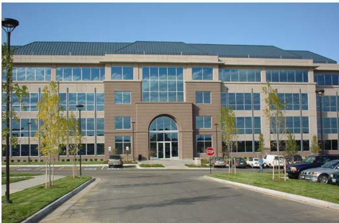
Main South Building
