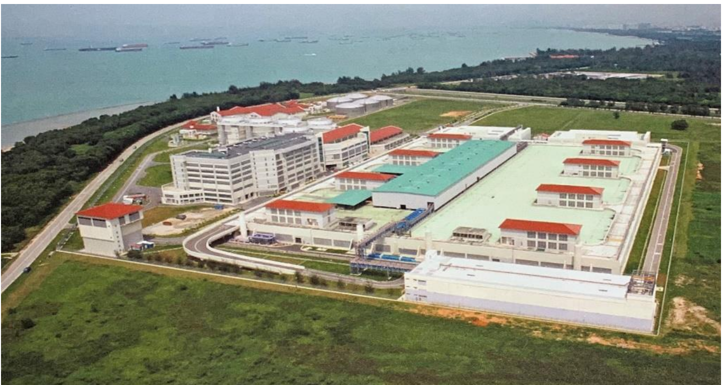
Changi Water Reclamation Plant, Singapore.
