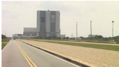
Back of the VAB, note the width for one of the crawler tracks is as wide as the two lane road
