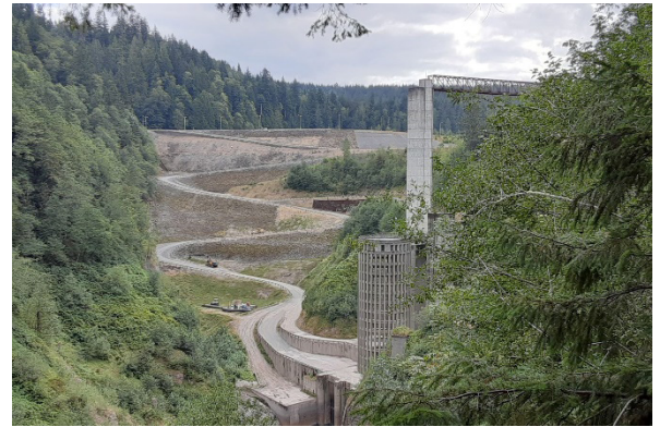
Mud Mountain Dam, upstream side.
