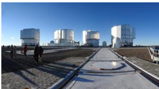
The VLT comprises four 8.2m fixed telescopes and four 1.8m moveable telescopes that travel on tracks in the foreground.
