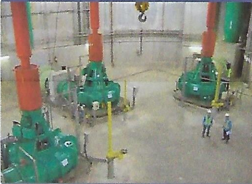
The completed pumping station
