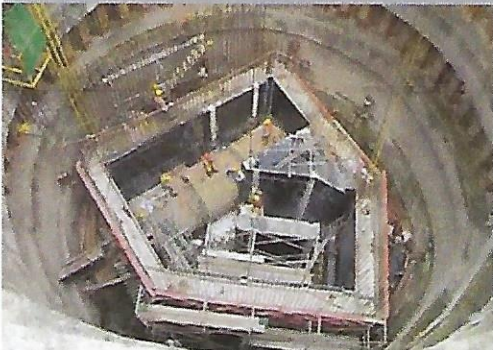
Construction of the deep tunnel sewer
