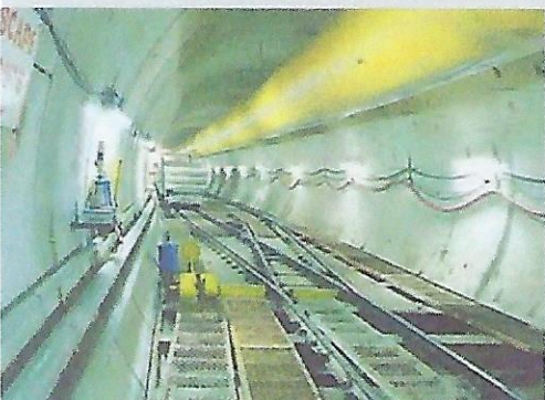
The completed tunnel
