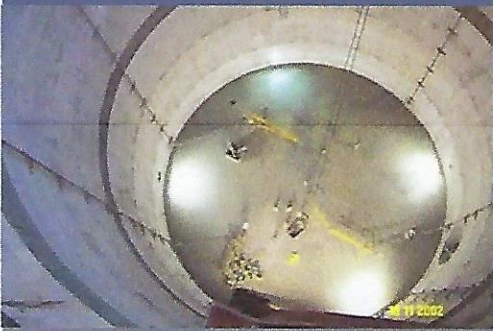
Construction of the deep pumping station
