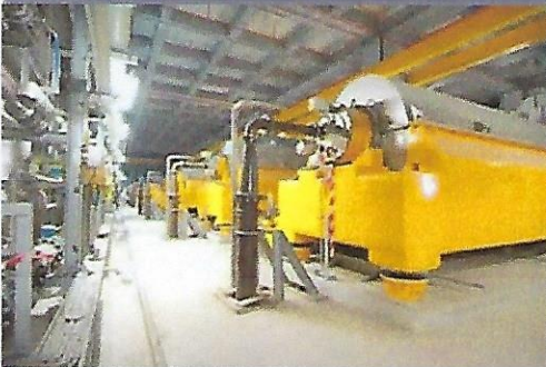
Thickening centrifuges
