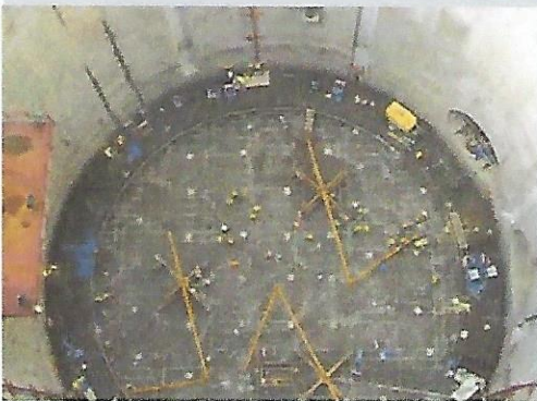
Pumping station construction
