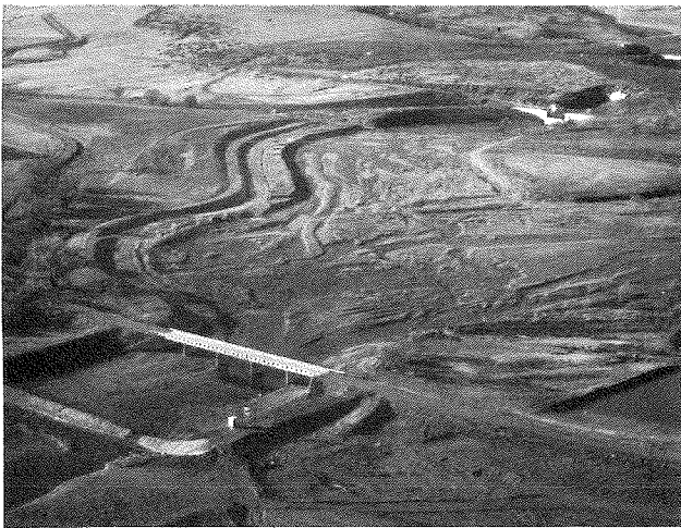
Tehama County Road P - 86.
