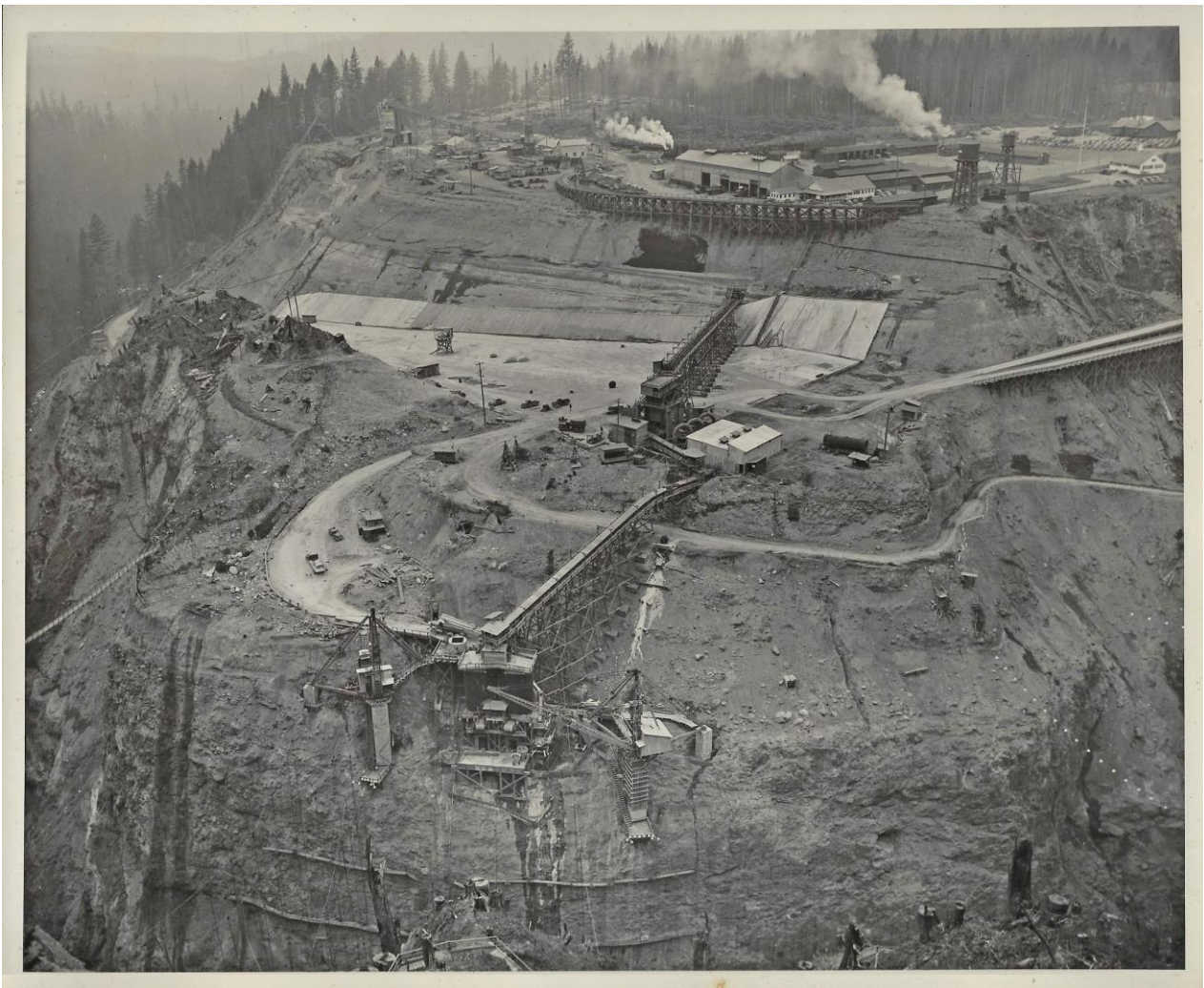
Progress view of the camp, spillway, and canyon wall.
