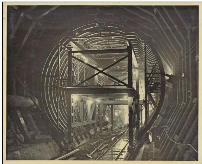
Steel forms for the concrete lining of the 23-foot tunnel.
