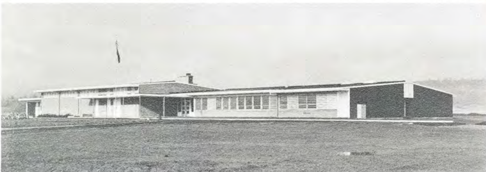
Garfield School, Corvallis, Oregon. Mechanical and electrical systems were designed for this elementary school. Jeppsen & Miller, AIA.
