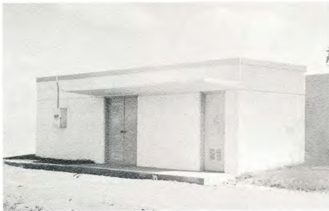
This pumping station at Nyssa, Oregon, is located over the caisson of a horizontal water collector having a capacity of 2.8 million gallons per day.
