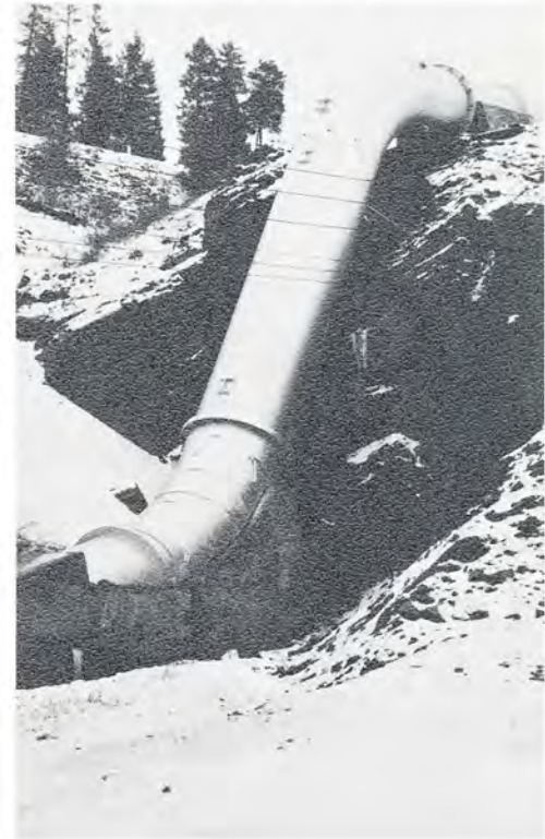
Steel penstock at Troy, Montana, for Montana Light & Power Company.
