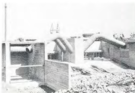
Pumped storage development.
