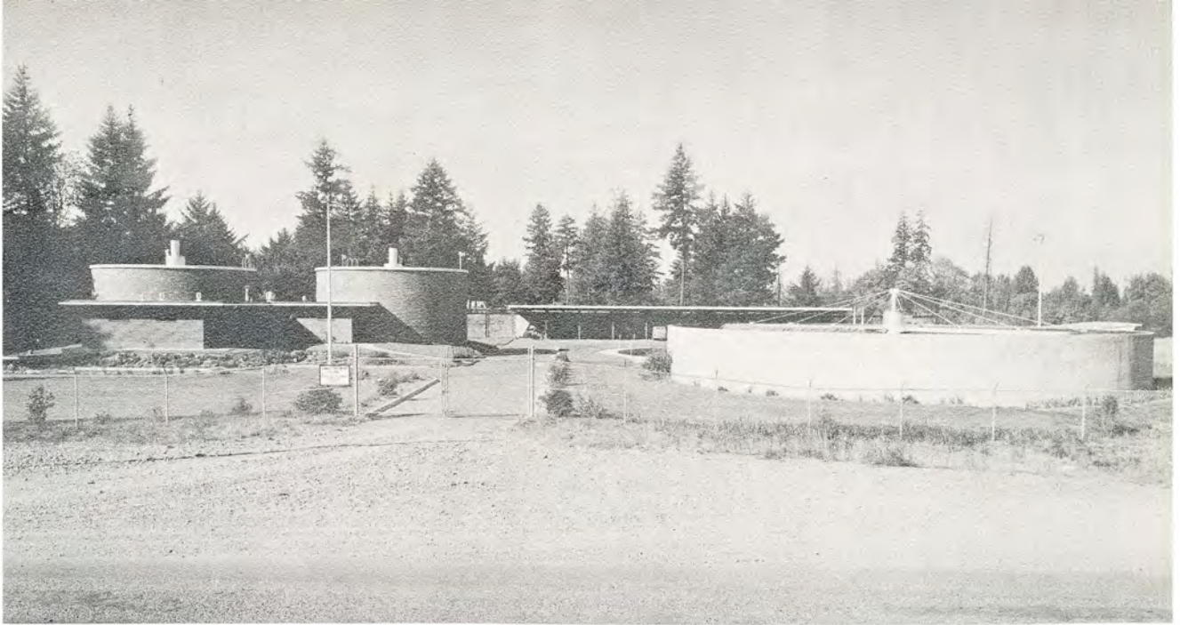
This Albany, Oregon, plant provides primary treatment with secondary facilities to handle industrial loads.
