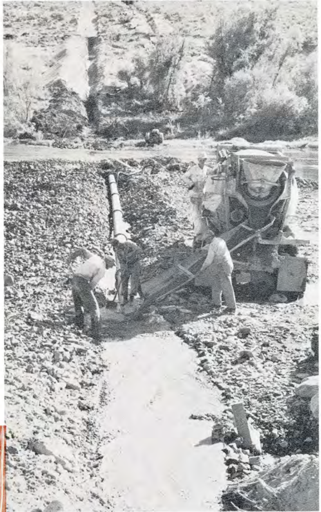
Installing water supply line across the Umatilla River. A successful river crossing must be skillfully planned and constructed under careful supervision.
