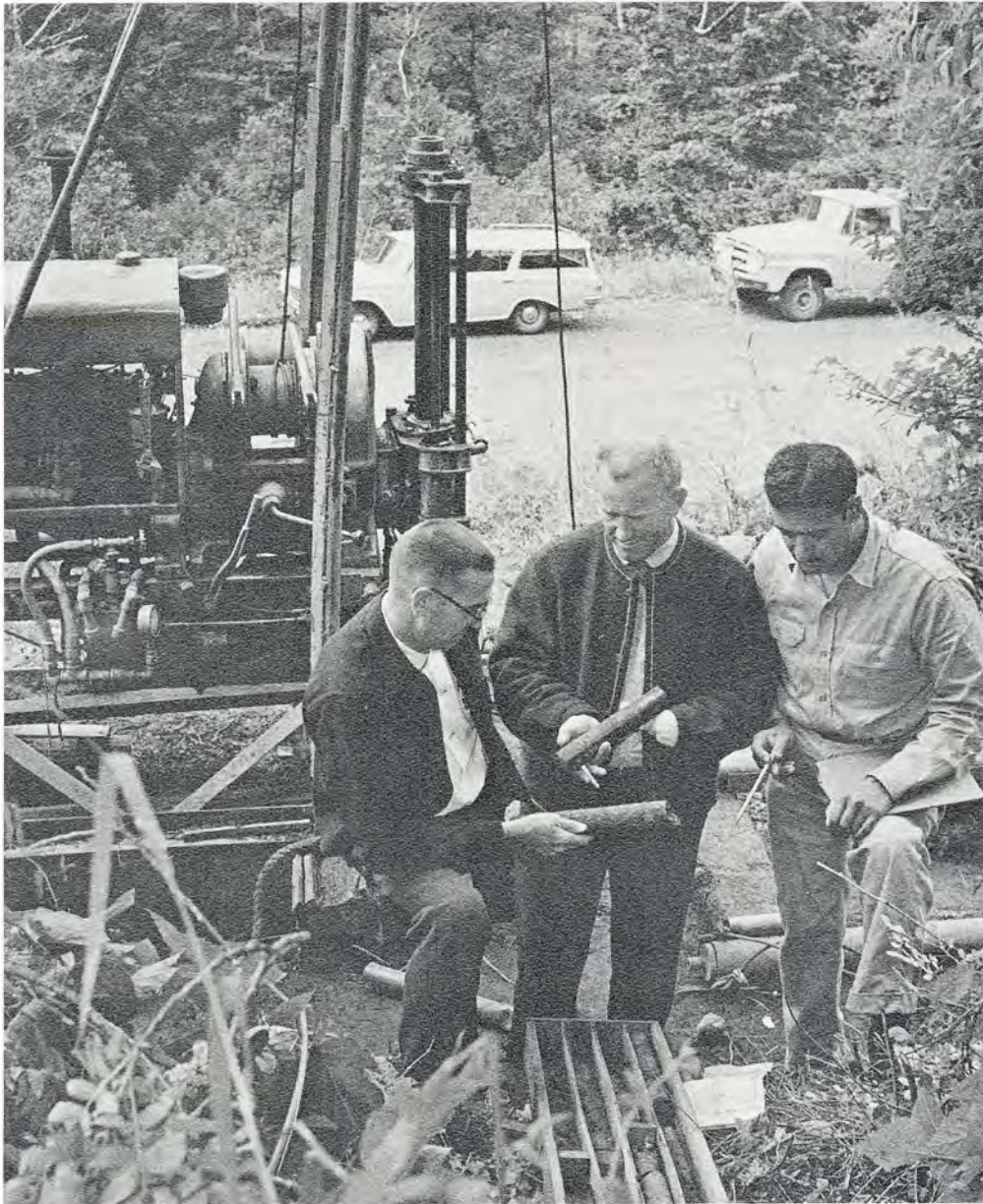
Extensive exploratory drilling operations were included in advanced planning study of the Trask River hydroelectric project for the Tillamook Peoples Utility District, Tillamook, Oregon.
