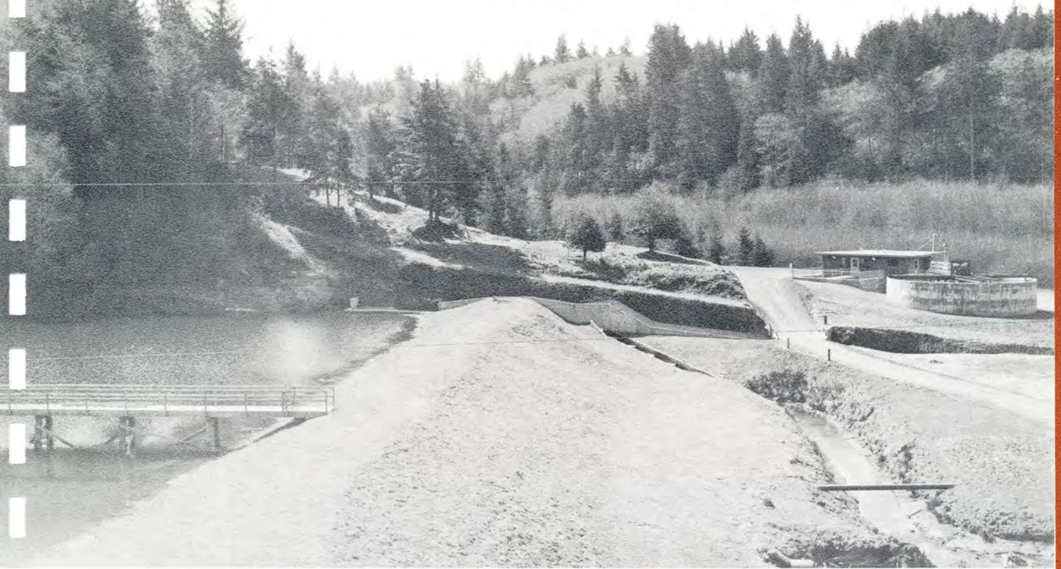
General view of the closely integrated water-storage and treatment-plant facilities at Newport, Oregon. Plant capacity is 1.5 million gallons per day.
