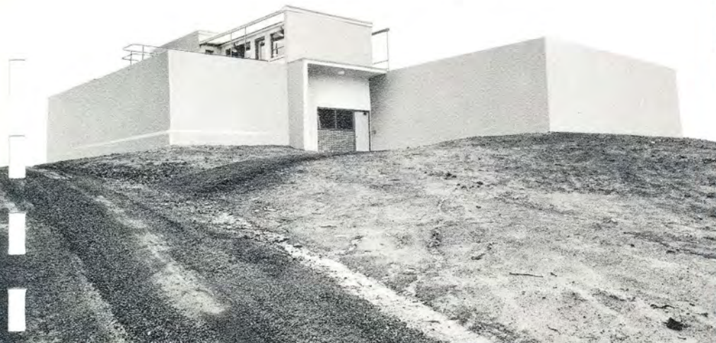
Coquille, Oregon, is served by this 1.5-million-gallons-per-day plant. Its hilltop location provides gravity feed to the city water system.
