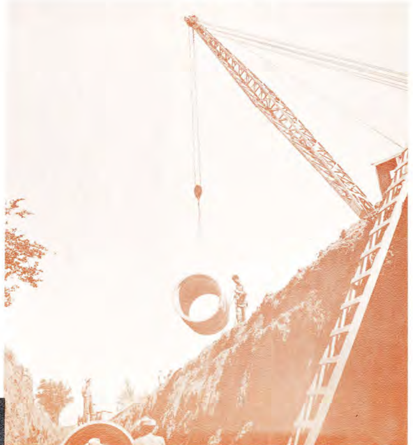
72-inch Interceptor Sewer, Eugene, Oregon.
