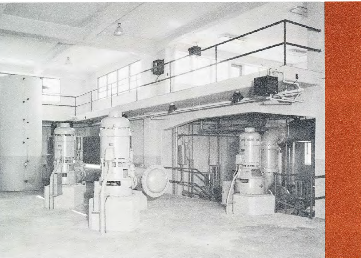
Pump room of the Corvallis Willamette River Plant. Plant design provides for economical expansion in increments to 16 million gallons per day. On its gravity supply system, Corvallis also has a treatment plant designed by this firm, with a capacity of 4 million gallons per day.
