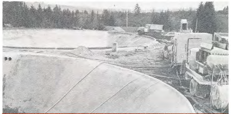
Repairing existing reservoirs at Dallas, Oregon.
