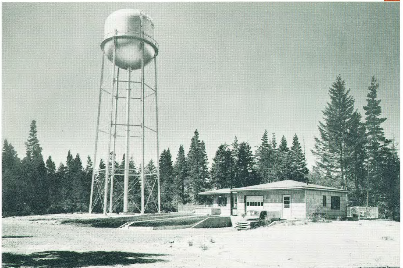
This compact, semi-automatic plant supplies 500,000 gallons of water a day for Florence, Oregon. The single location for reservoir and plant virtually eliminates clearwell cost.
