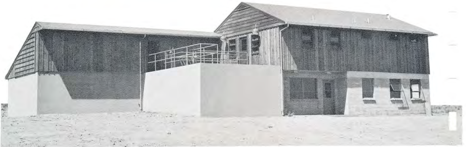
Madras, Oregon, now has a modern 600,000-gallons-per-day water-treatment plant. Special problems resulting from severe climatic conditions and raw water of poor quality were solved.
