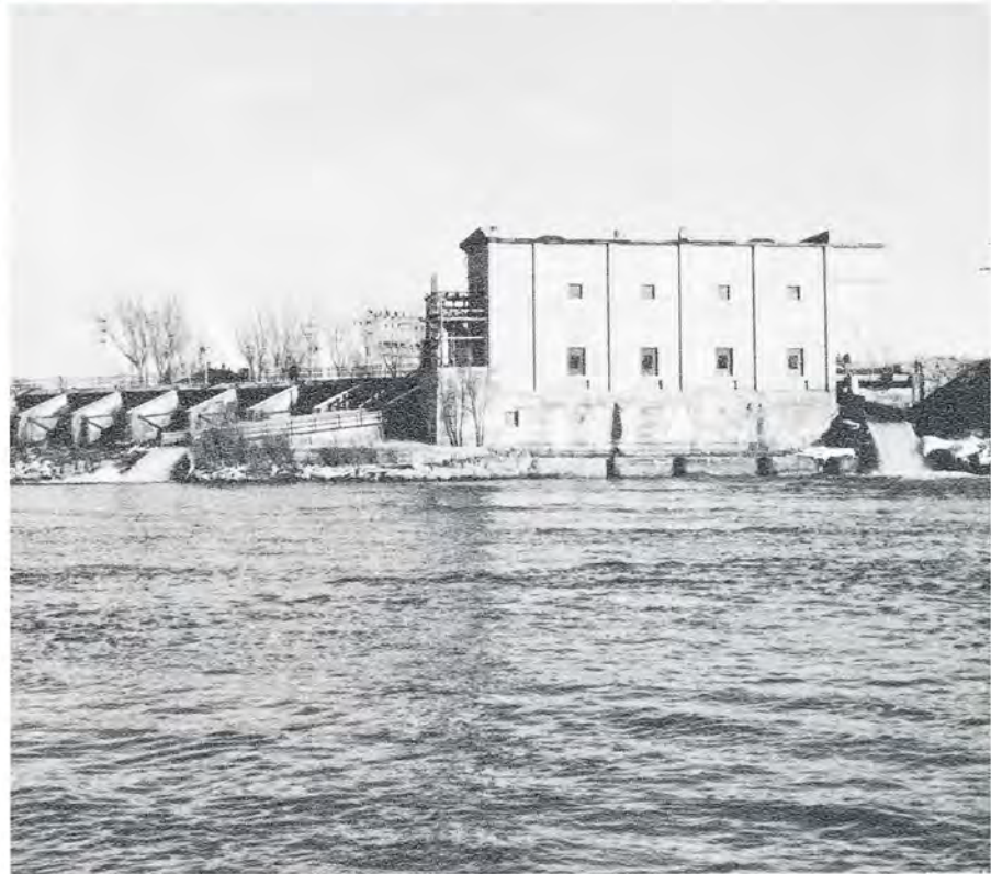
Supervisory control system for operation from a central control room was designed for the 3,000 KW Lower Hydroelectric Plant of the City of Idaho Falls, Idaho. Other work included design of repairs and renovation for the powerhouse and spillway structures.
