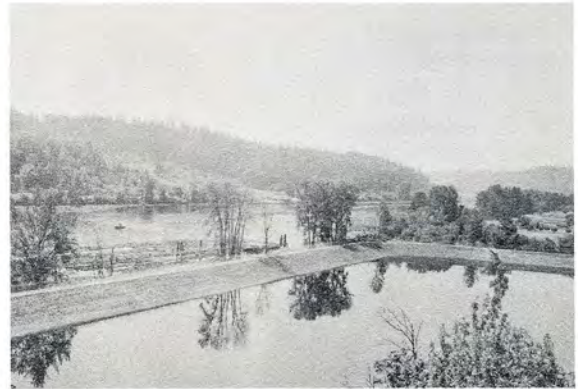
A serious industrial waste problem was solved by the construction of this 90-million-gallon sulphite-liquor storage lagoon for the Crown-Zellerbach Corporation at West Linn, Oregon.
