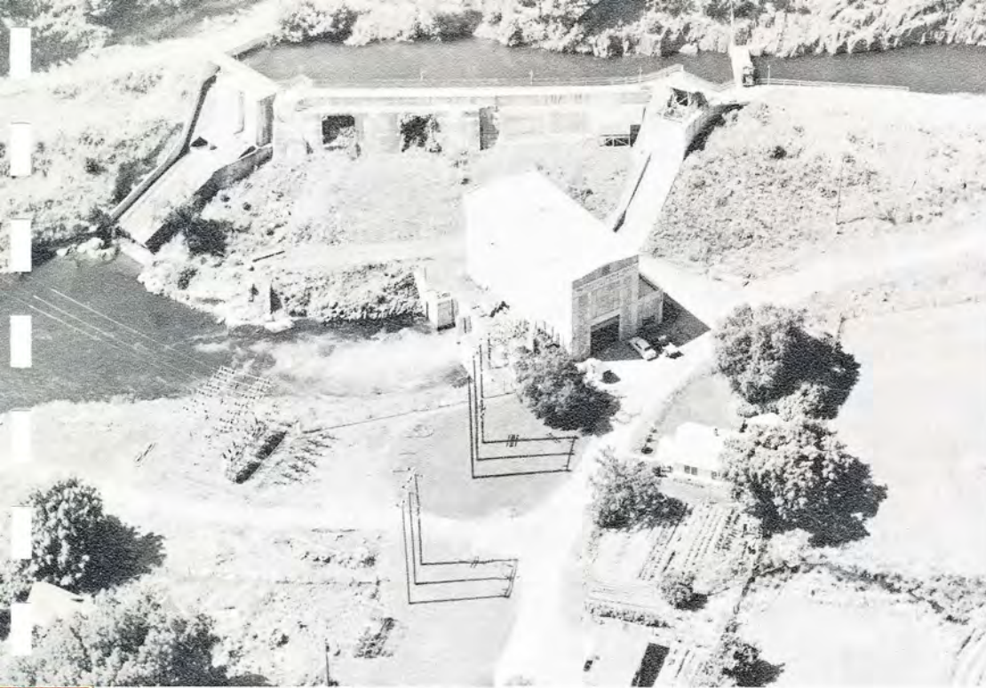
Aerial view of Walterville hydroelectric station.
