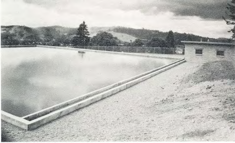
2.3-million-gallon reservoir and chemical-feed building at Cottage Grove, Oregon.
