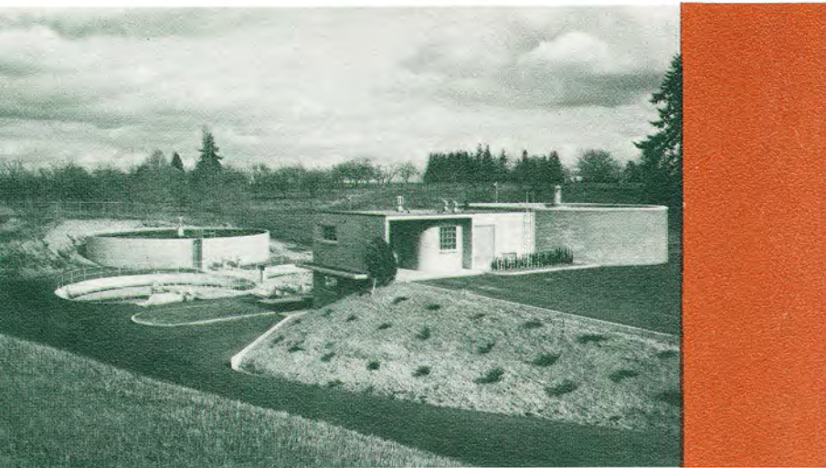
This attractive plant at McMinnville, Oregon, utilizes a difficult gulch site.
