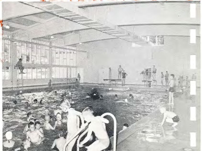
Swimming Pool Reedsport, Oregon Wilmsen & Endicott, Building Architects
