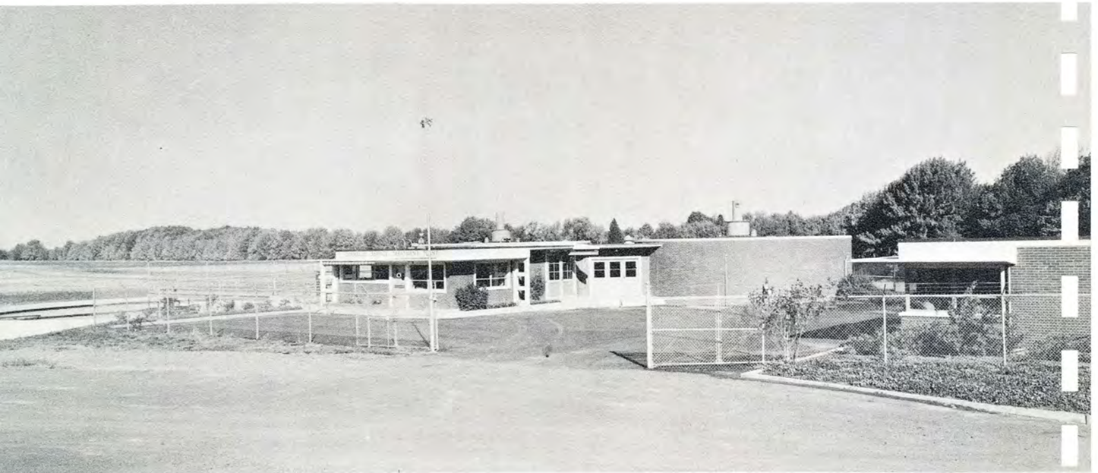
Primary sewage-treatment plant at Corvallis, Oregon.
