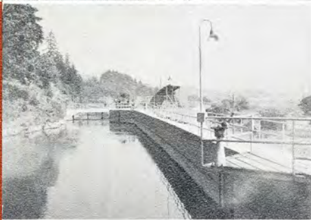
Forebay. Racks and penstock gate in background.
