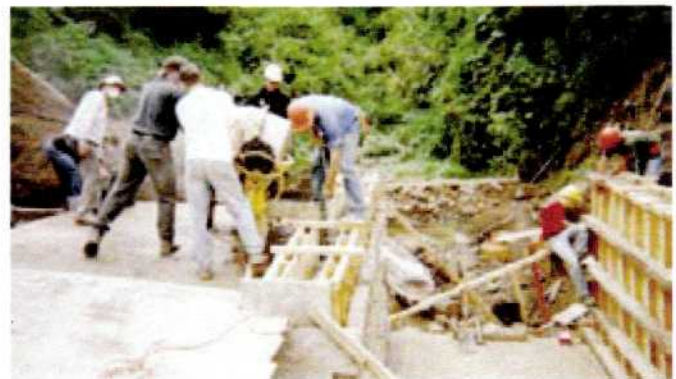
Marquette University students construct a bridge in Guatemala.
