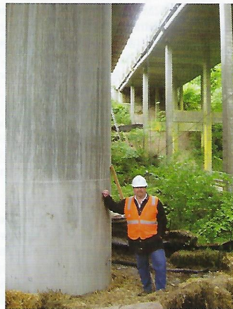
Designing and installing the bridge foundation in less than perfect soils is one of the project’s toughest challenges.
