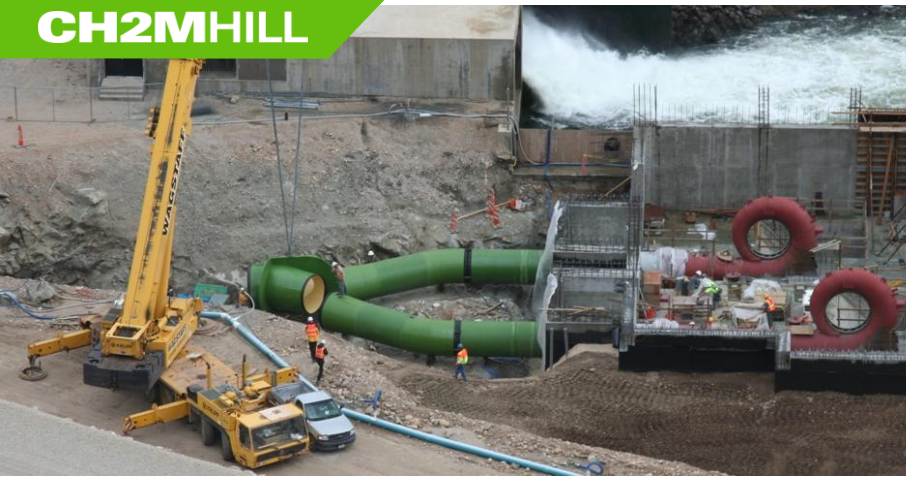
Jordanelle Hydro Project for the Central Utah Water Conservancy District
