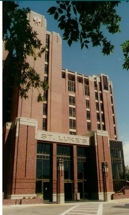
St. Luke's Regional Medical Center – East Tower Expansion
