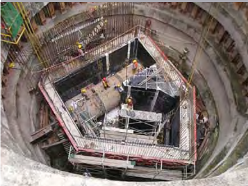
Construction of the deep tunnel sewer
