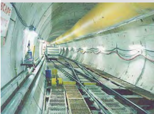
The completed tunnel
