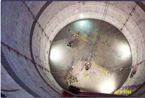
Construction of the deep pumping station
