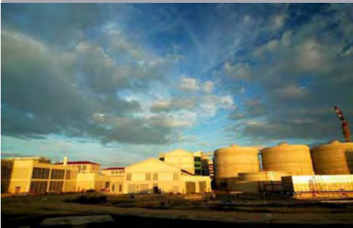
The Changi water reclamation plant at sunset
