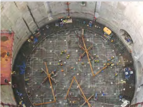
Pumping station construction
