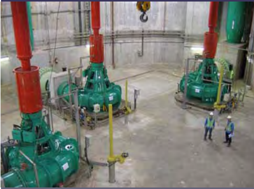
The completed pumping station
