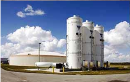
Equalization basin (left) and odor control facilities (right) at the East Water Reclamation Facility
