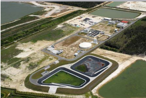
Aerial view shows BSU facility, stormwater pond, rejects pond, reclaimed water storage ponds, and area for future expansion
