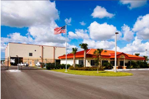
Ops building and entrance to BSU's state-of-the-art East Water Reclamation Facility.
