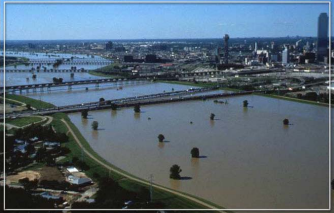
View of the flooded Trinity River in 1990. Here the river nearly fills the entire 2,000-foot-wide floodway
