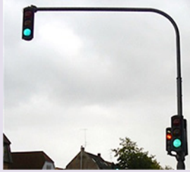
Bicycle and auto traffic lights. The big light is for cars, etc. Green is go; the little red light next to the bottom big light is for bicycles.
