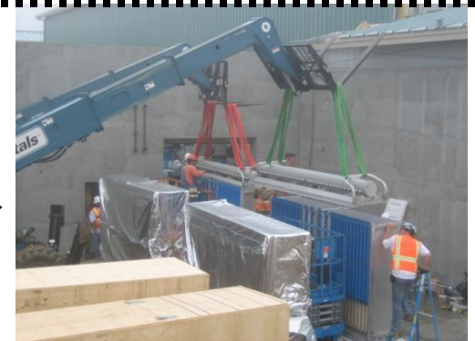
Cassette uncrating and header installation - Nov '07
