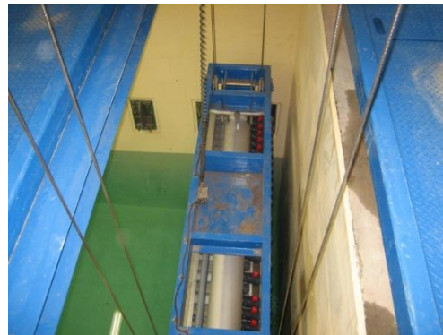
Cassette install in tank - Nov '07
