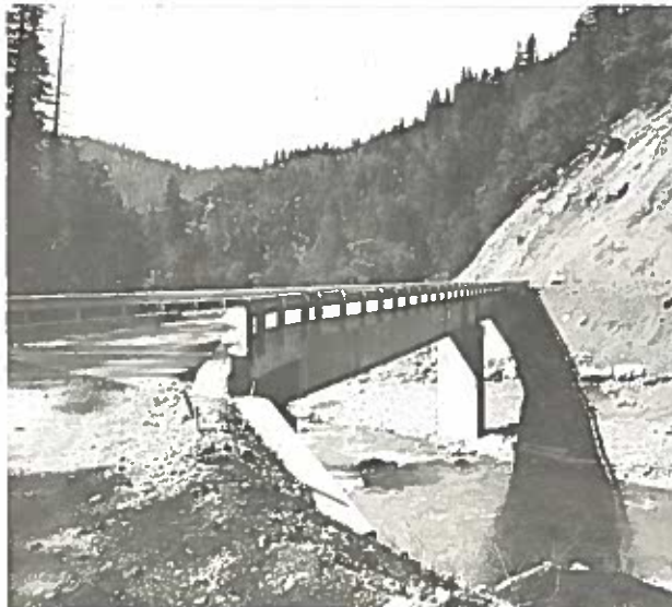
New River Bridge U. S. Forest Service Shasta-Trinity National Forest
